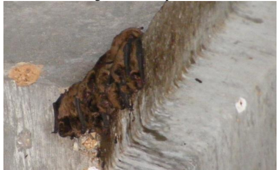
Big brown bat cluster day roosting under bridge
