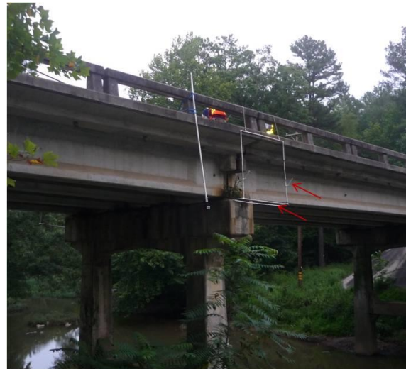
Figure 4. Net with bottom shelf and weighted spurs suspended over the bridge at the expansion joint. Note that the shelf effectively brought the bottom of the net closer to the opening, though the spurs did not provide the desired effect.
