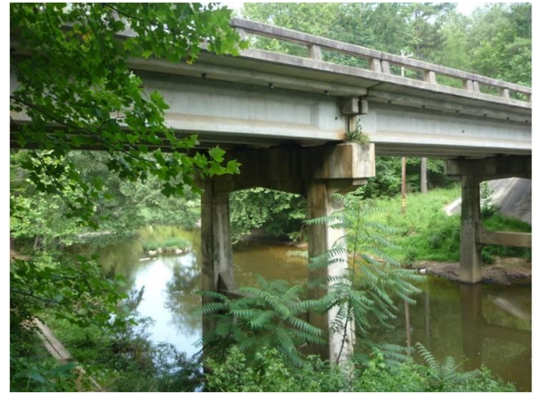
Figure 1. Expansion joint on Cole Mill Road Bridge over the Eno River, Durham County, NC. Arrow indicates location of emergence.
